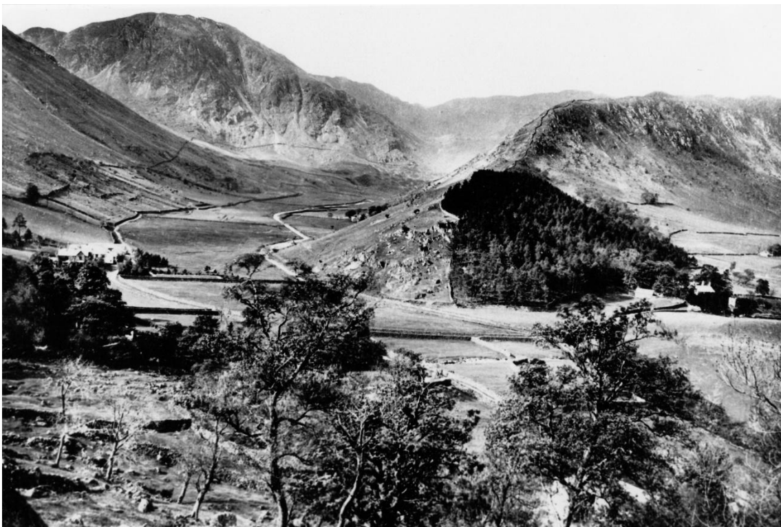
Figure 72: Mardale of old A peaceful valley head; tiny church; friendly inn; tranquil scenery
