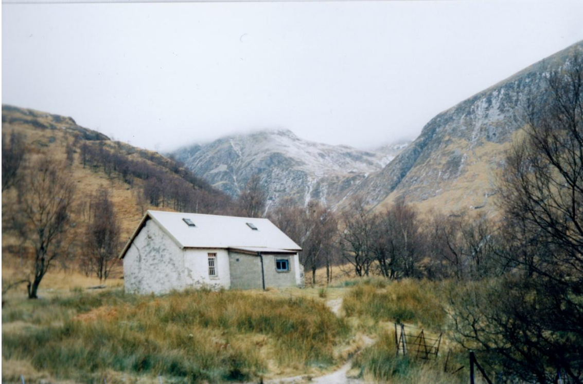
Figure 41: Mountain rescue hut Steall
