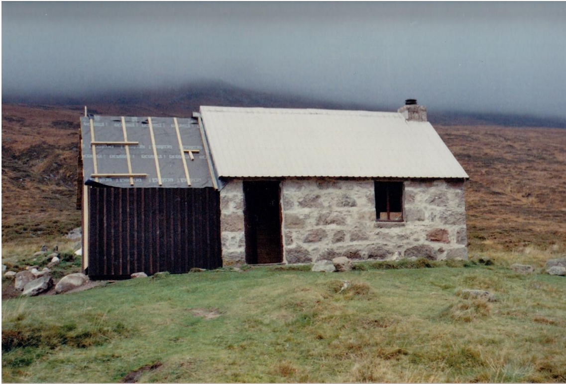
Figure 2: Corrour bothy in the process of upgrade
