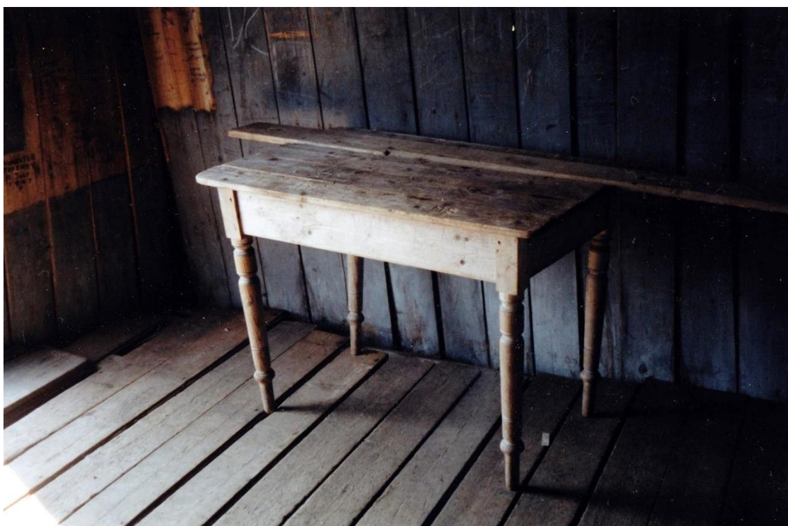
Figure 21: Tin bothy on slopes of A'Chailleach - interior view How long will this stand?
