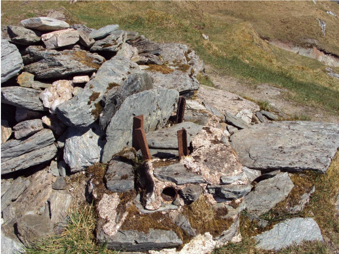
Figure 70: Beinn Bhuidhe collapsed trig. column
