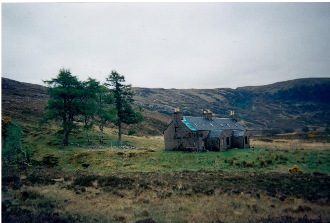
Figure 30: Renovation at Achneigie
