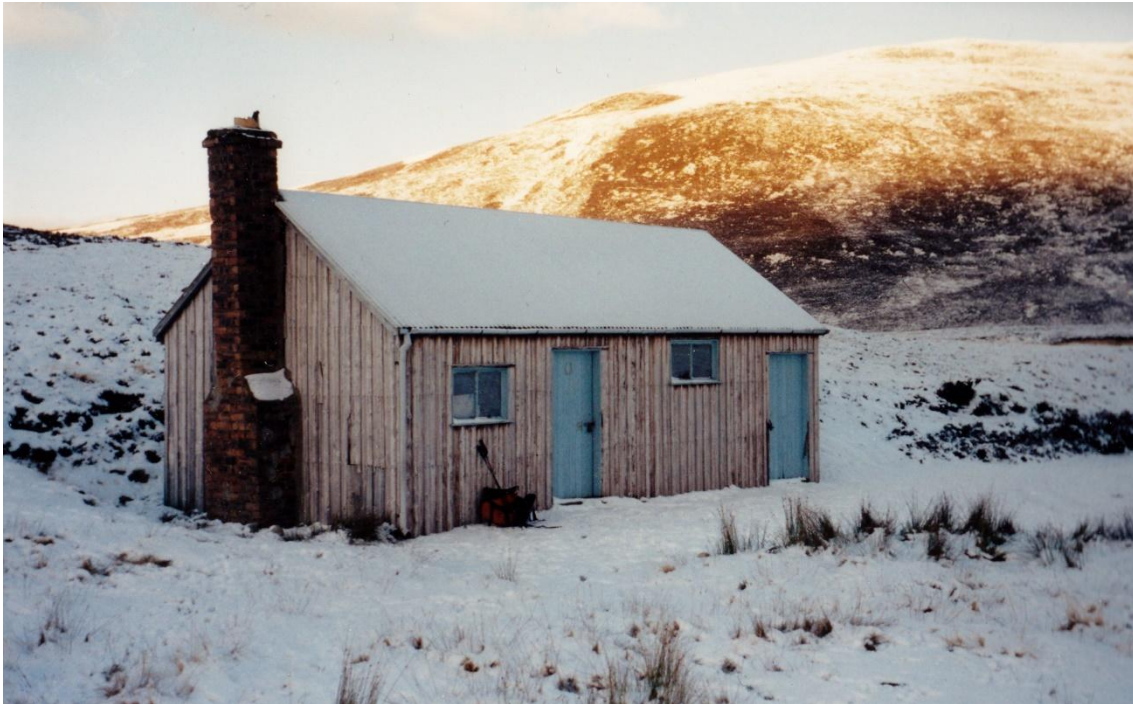
Figure 44: The private locked bothy on the banks of Loch Cuaich
