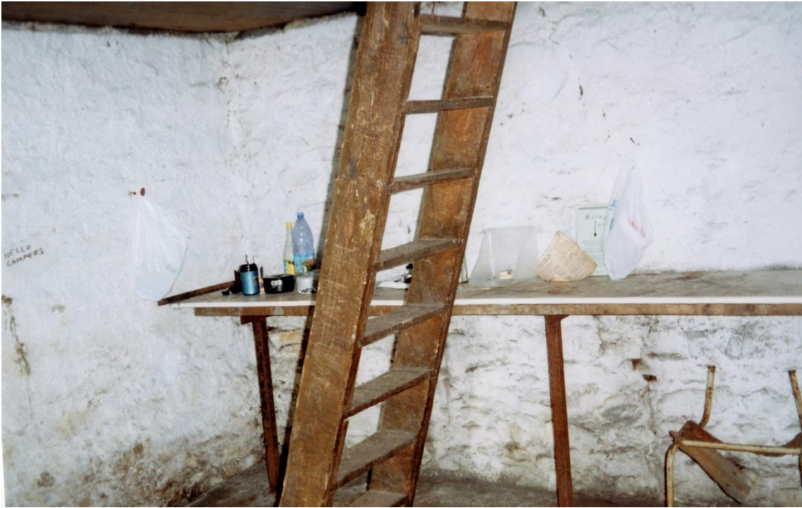
Figure 11: The steep steps leading to the attic at Lairig Leacach
