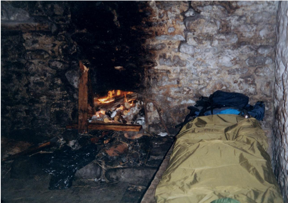
Figure 5: The warm end of Corryhully bothy
