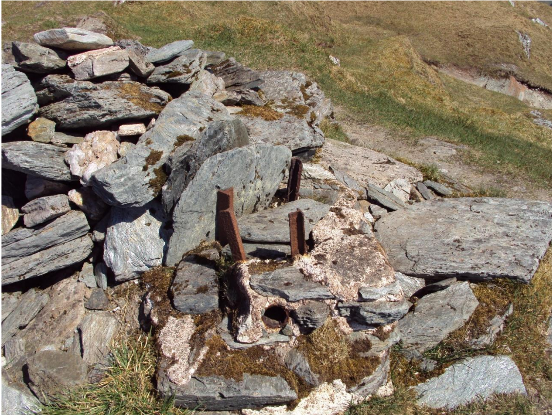
Figure 70: Beinn Bhuidhe collapsed trig. column
